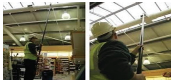
Fig. 2: Conventional Under Roof Cleaning
