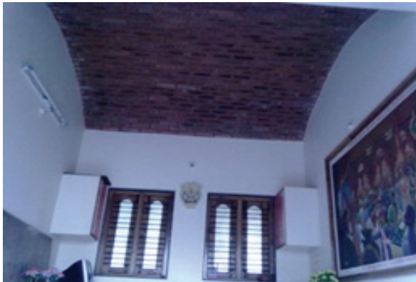
Fig. 3: Brickwork Roof top
