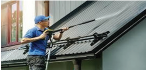
Fig. 4: Roof cleaning with a water jet
