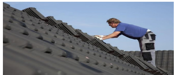
Fig. 3: Climbing on the roof
