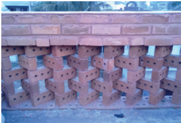
Fig. 5: Brick Parapet on Terrace
